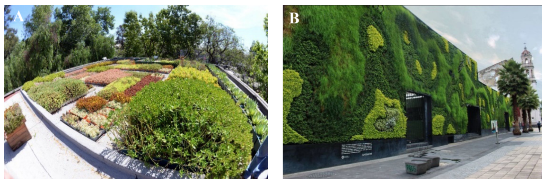
Figure 1. A: Extensive green roof; B: Outdoor green wall.
